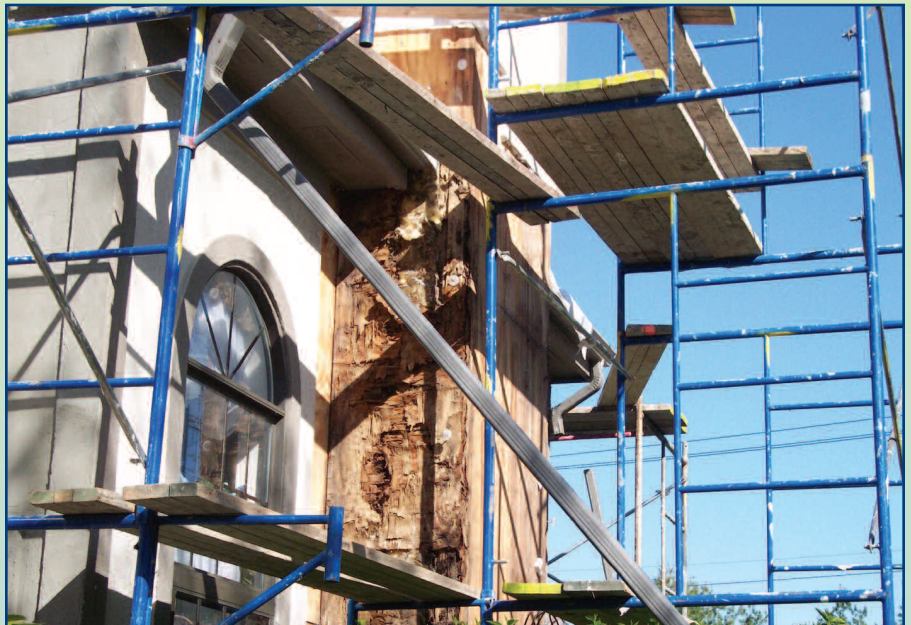
Example of EIFS removal during repair process.
